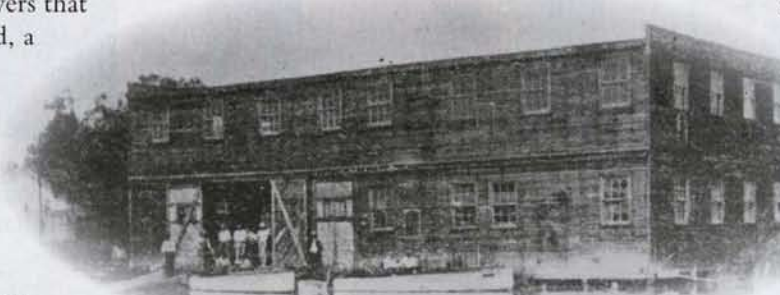
CRAFT MAKER Starting in 1911, founder Louis Mayea operated from this wood structure in Fair Haven, Mich.
